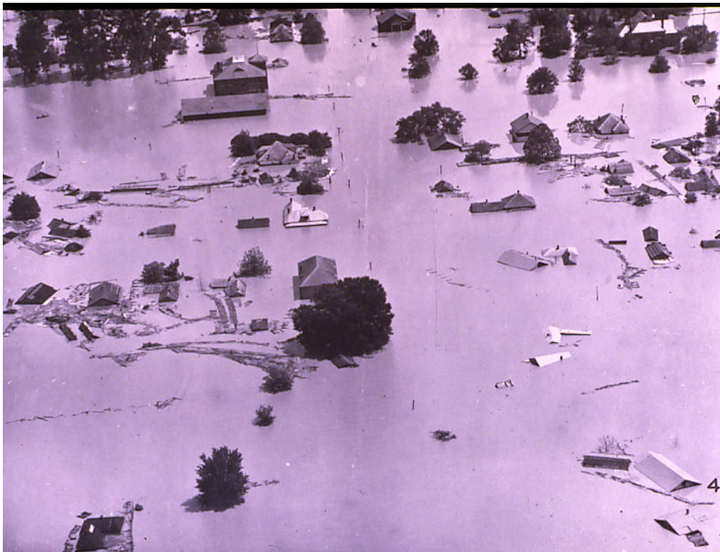
Arkansas City, 1927 flood
