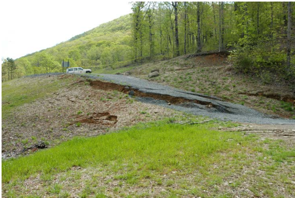
Figure 13. Ground displacement and subsidence east of the Bradford house.
