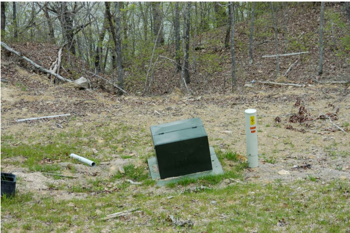
Figure 19. Phone and power boxes displaying effects of subsidence and displacement marginal to main slide area.
