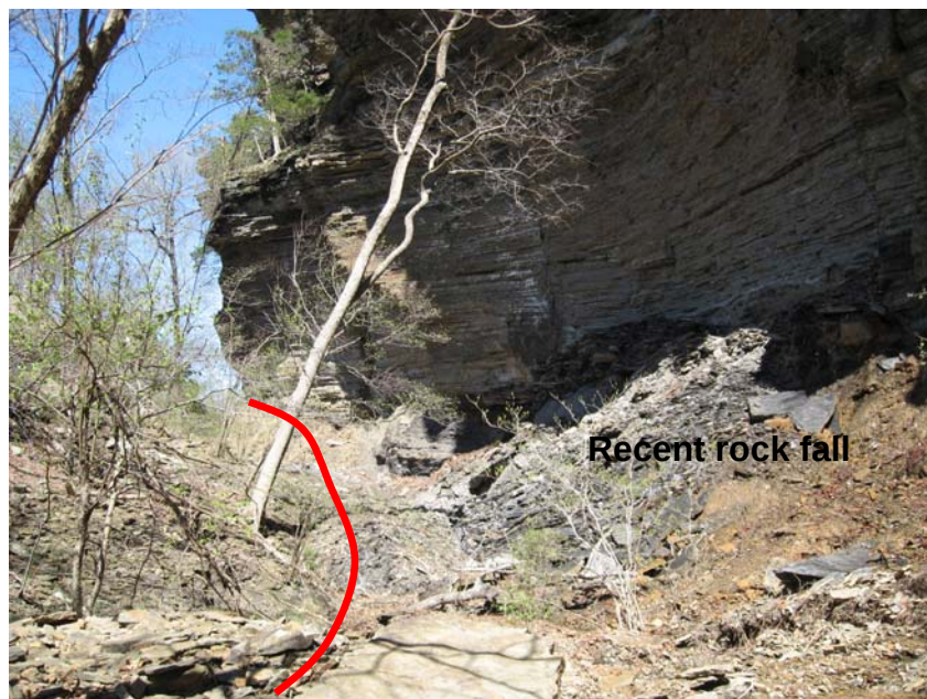
Cane Hill bluff over which several waterfalls probably poured over onto shaly interval. Red line shows head of old slide scarp.
